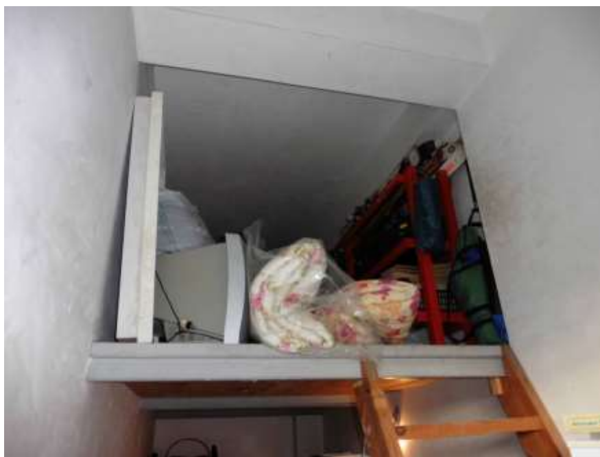
Foto 4 – Garage “9A” – Soppalco
