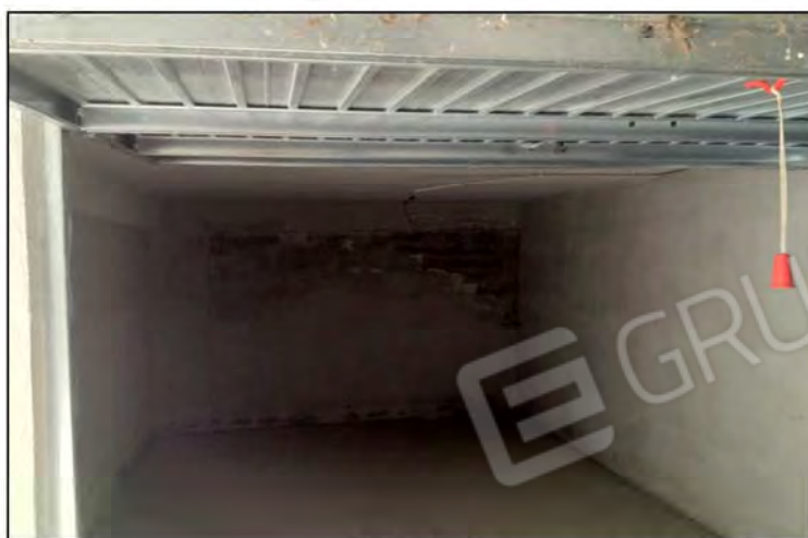
(Foto 6 – Box garage – Part. n°974, Sub 20)
