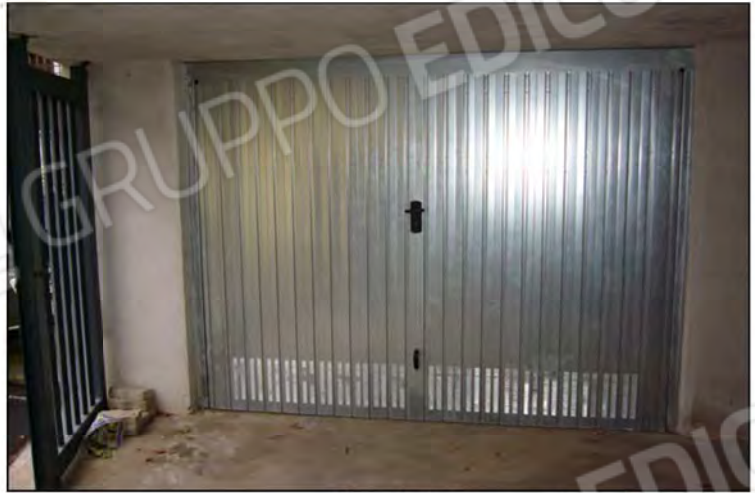
(Foto 7 – Box garage – Part. n°974, Sub 19)
