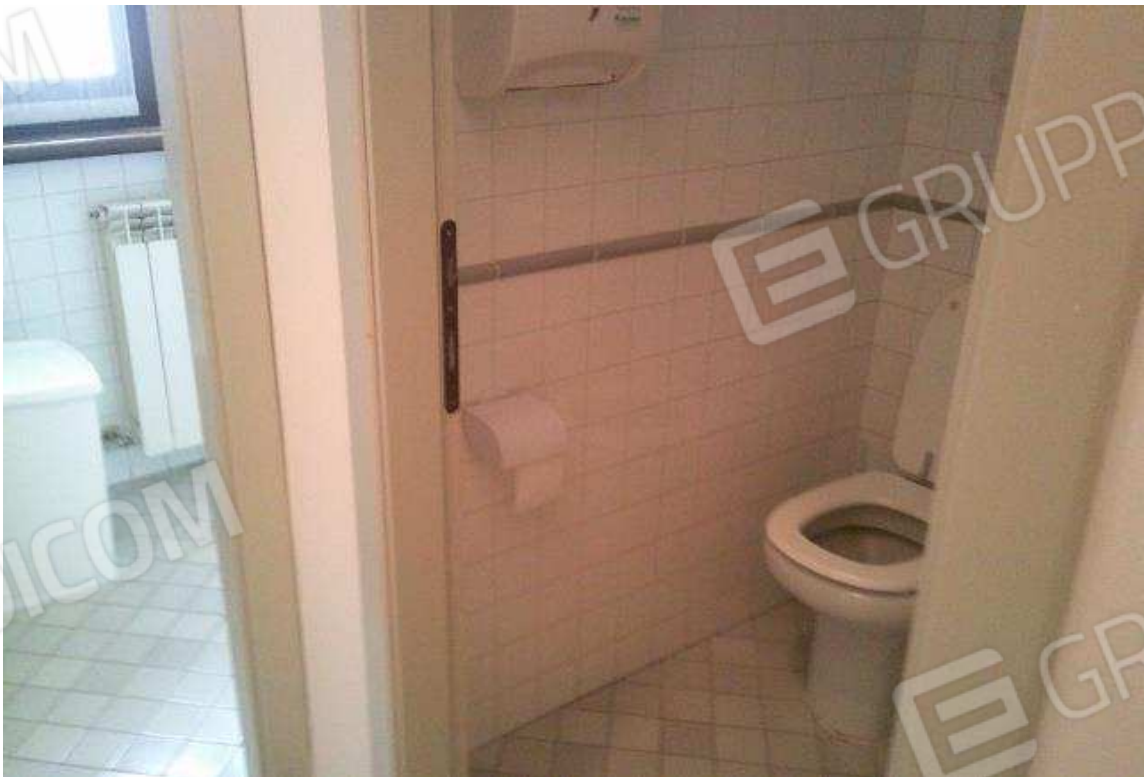
VISTA BAGNO SUB. 36
