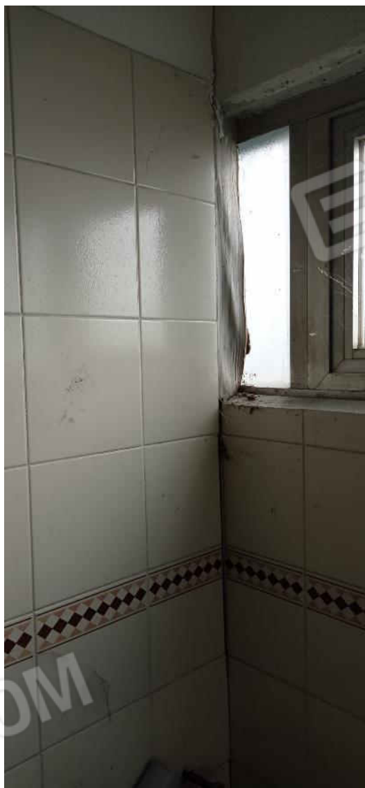
73-bagni piano terreno
