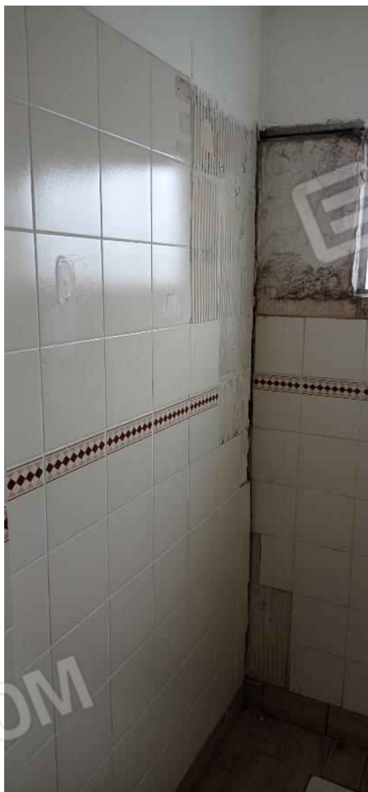
77-bagni piano terreno
