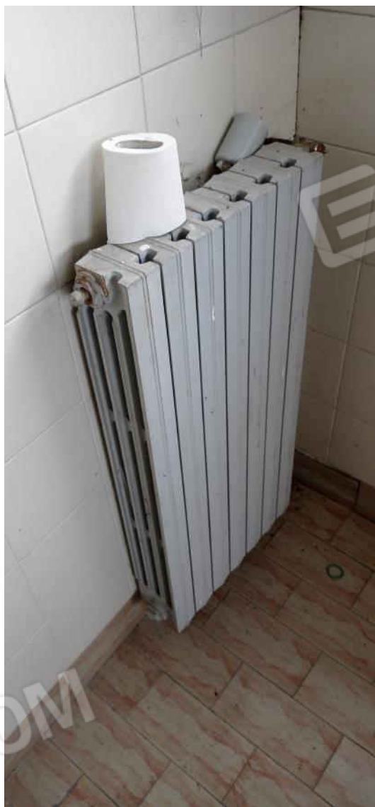
75-bagni piano terreno
