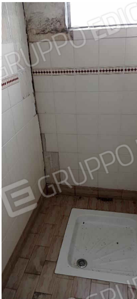
74-bagni piano terreno
