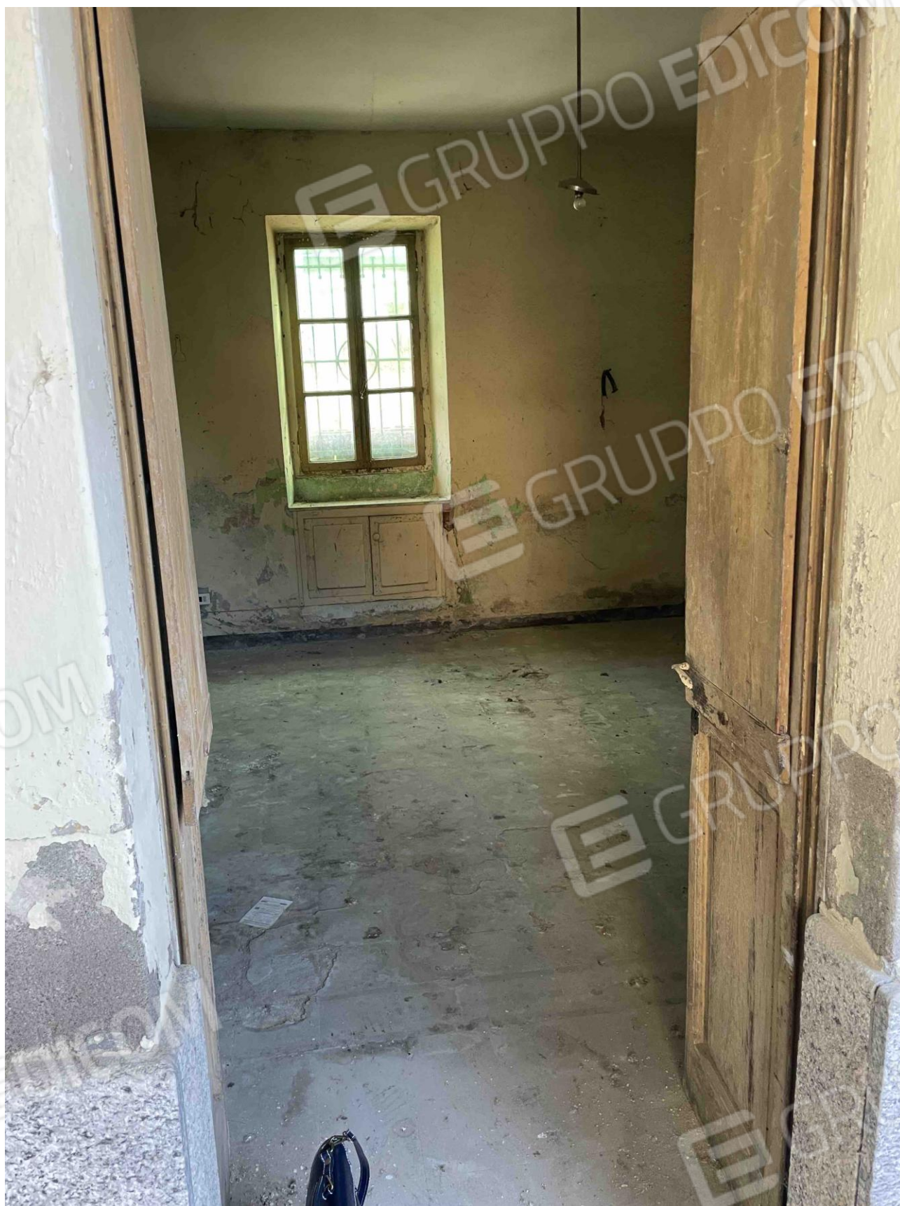
LOCALE SGOMBERO PIANO TERRA
