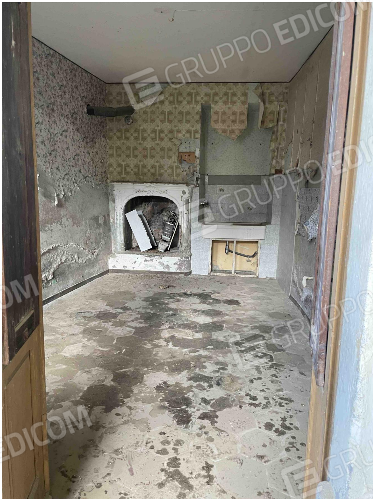
LOCALE PIANO TERRA
