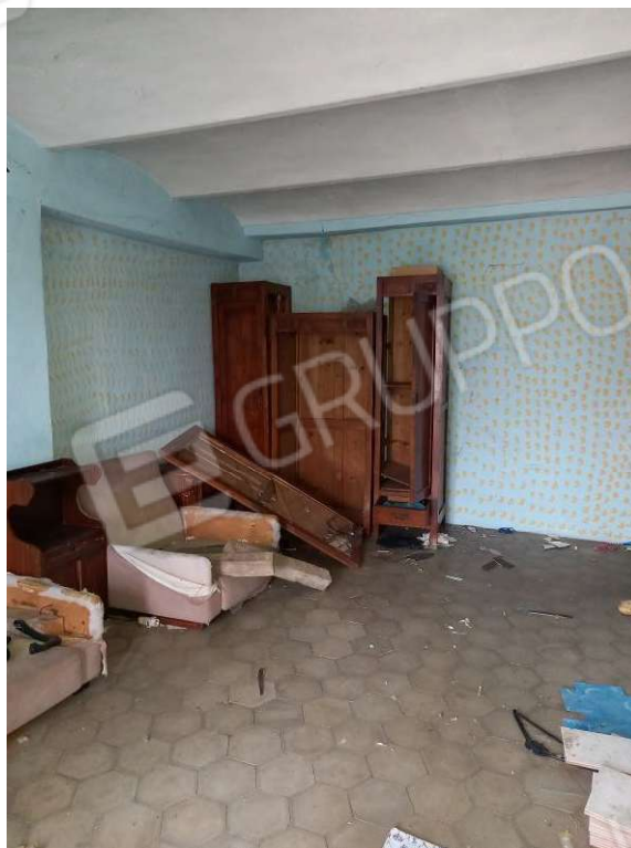
Vista interna locale Camera 1
