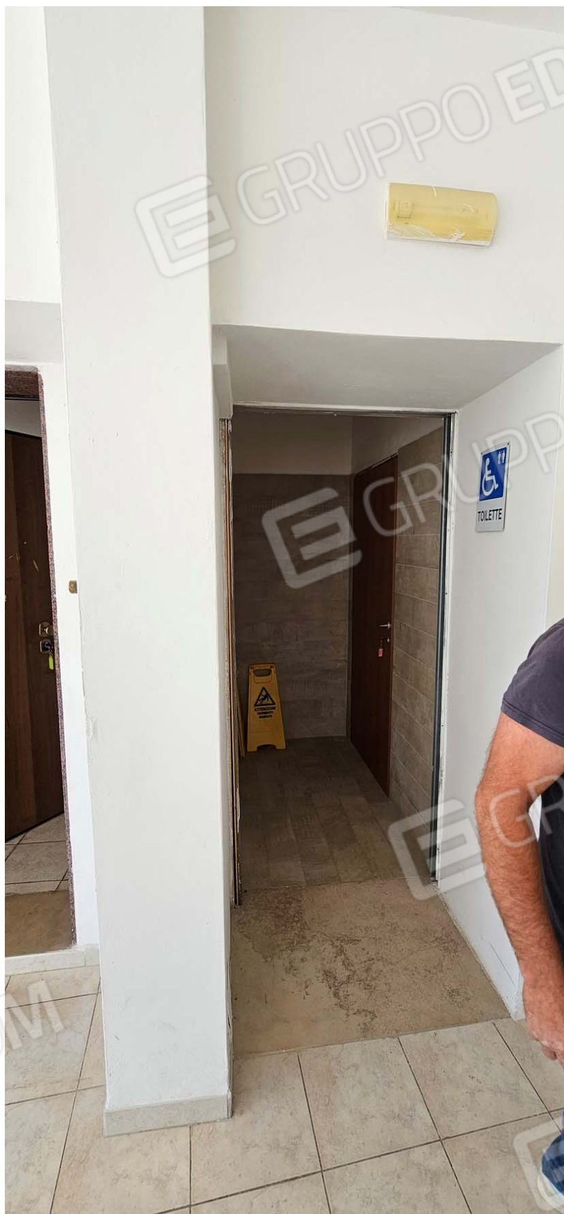
Vano difforme: bagni piano terra
