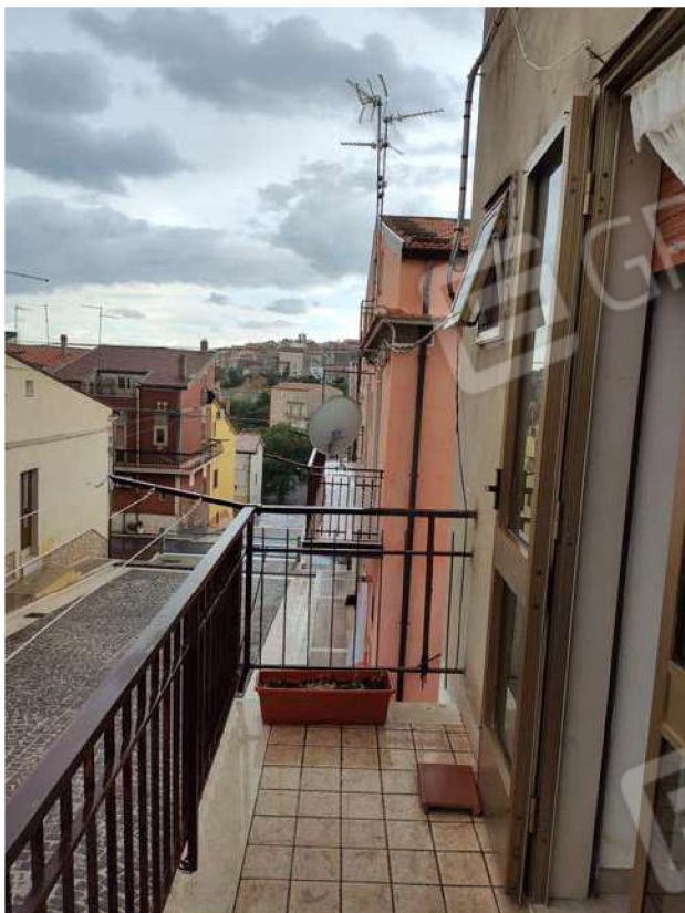
Sub. 4 – Balcone [Foto 16]
