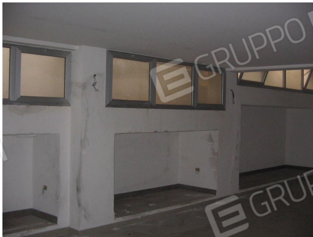
Locale – piano interrato
