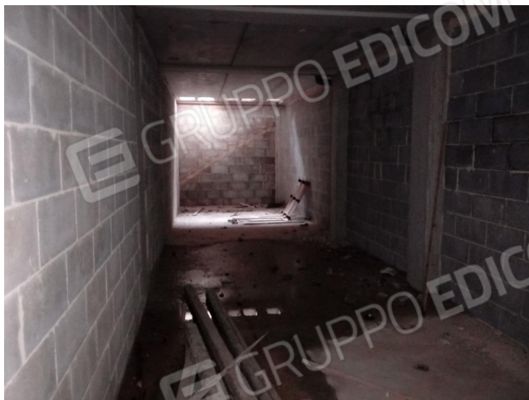
Locale – piano interrato
