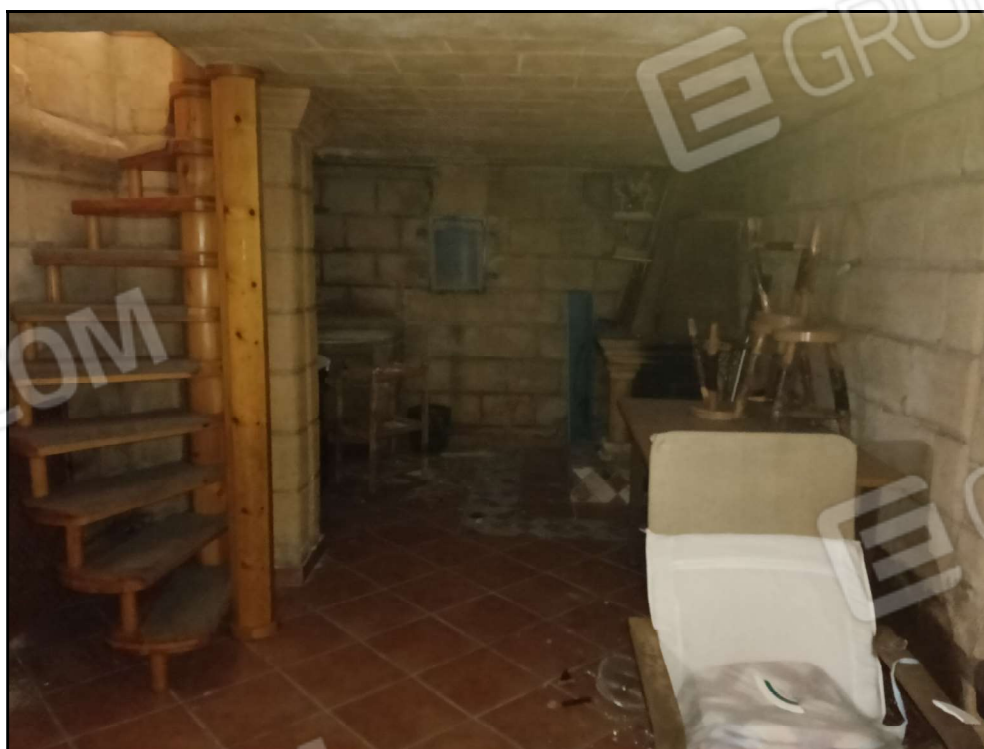
Fot. 2 – Piano interrato–
