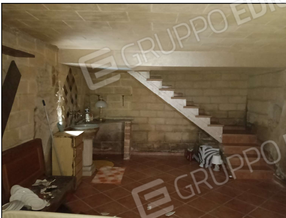
Fot. 3 – Piano interrato –
