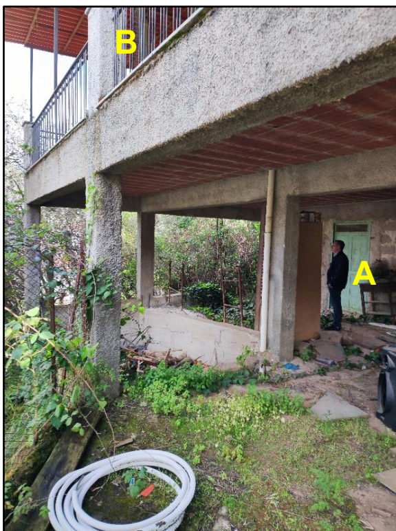
(A) Piano seminterrato - (B) Balcone coperto al Piano terra
