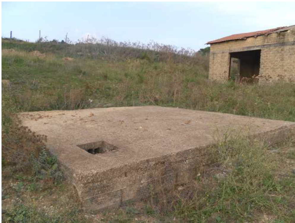
Cisterna particella 170 sub 1
