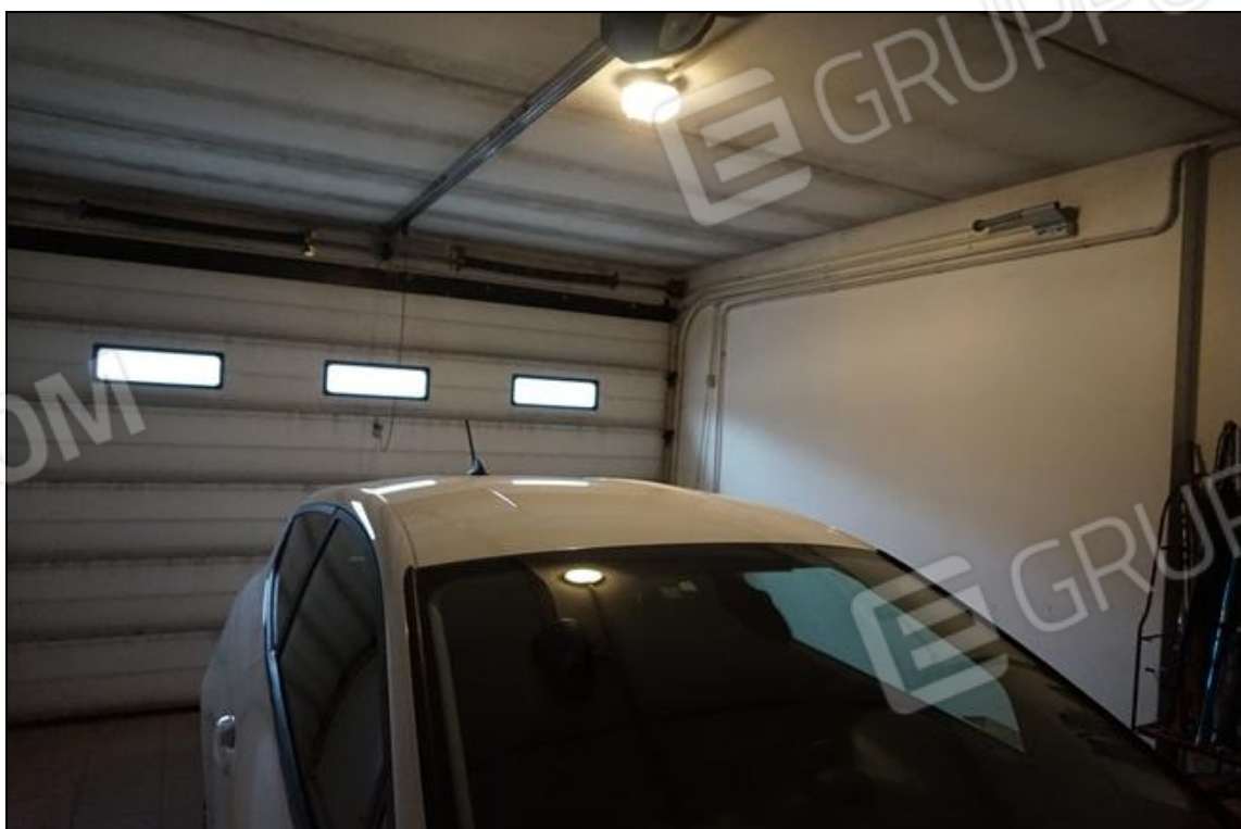
FOTO 38 – Piano interrato – Garage sub.46
