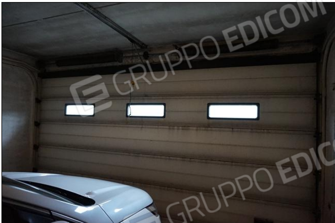
FOTO 37 – Piano interrato – Portone garage sub.45
