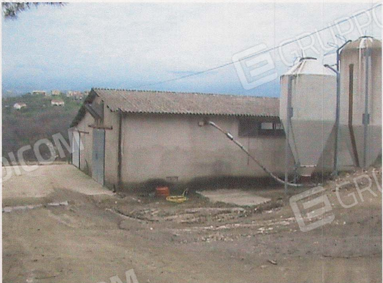
6. CAPANNONE AGRICOLA FOLIO 38, PART. 392
