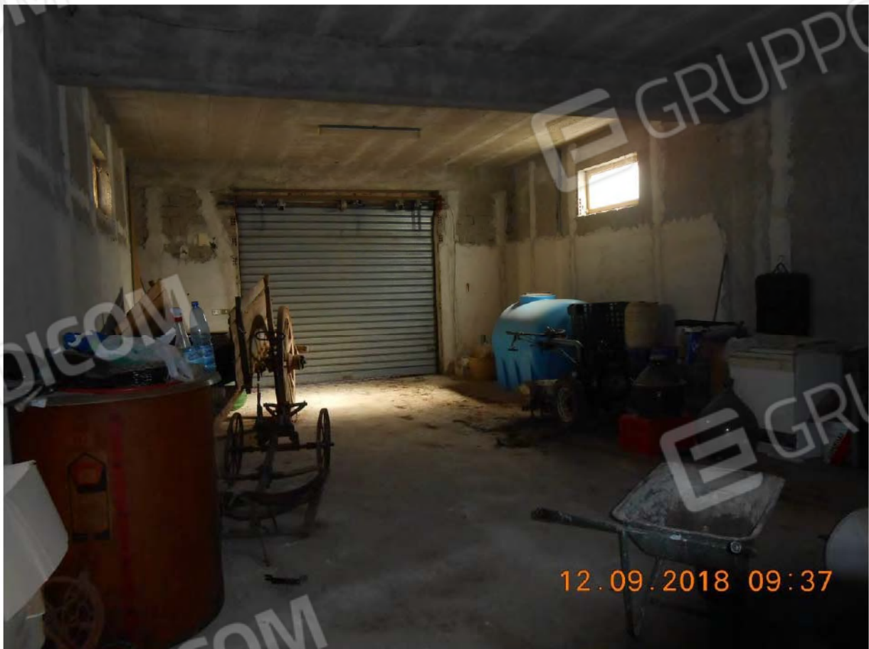
Foto 4. Garage – piano terra
