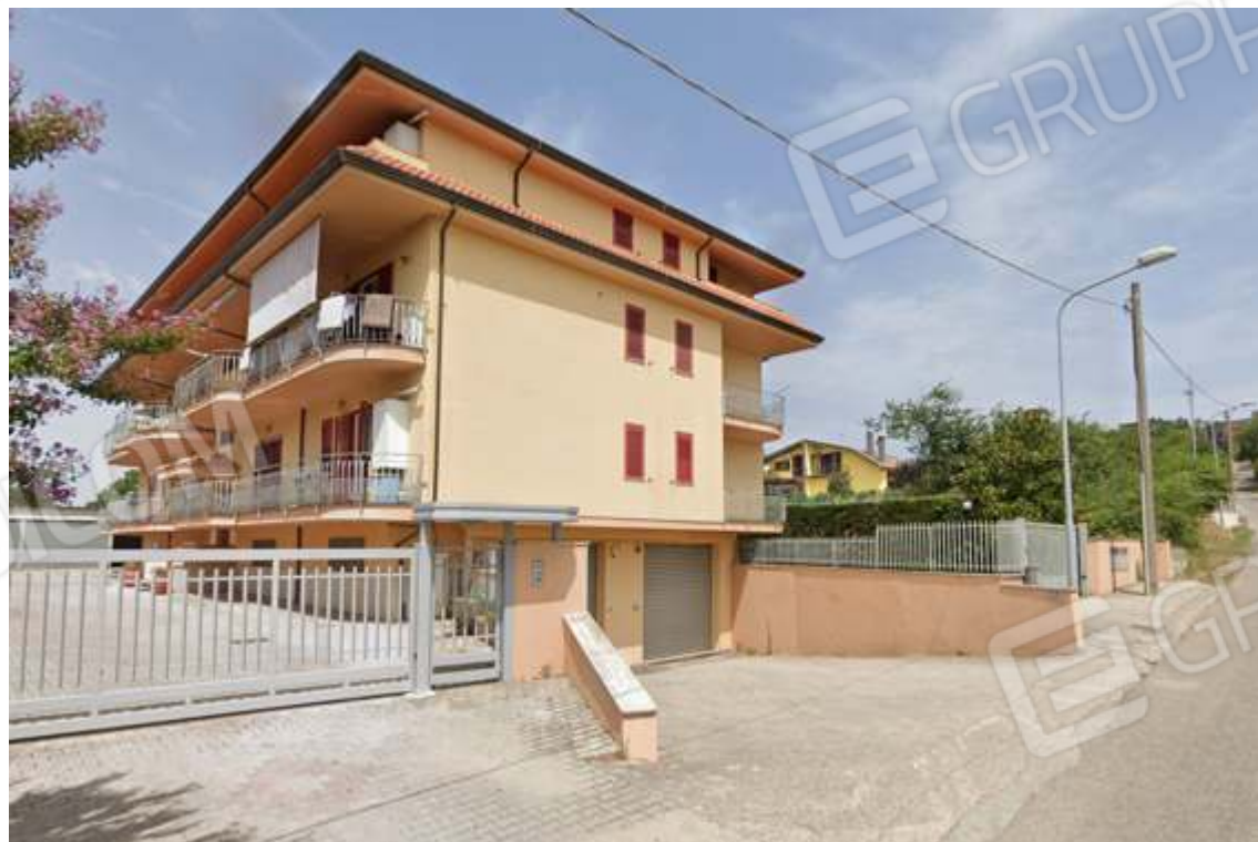
Fig.2 – Vista dell’immobile da via Ciesco Porrelle (fonte Google Maps 2021)
