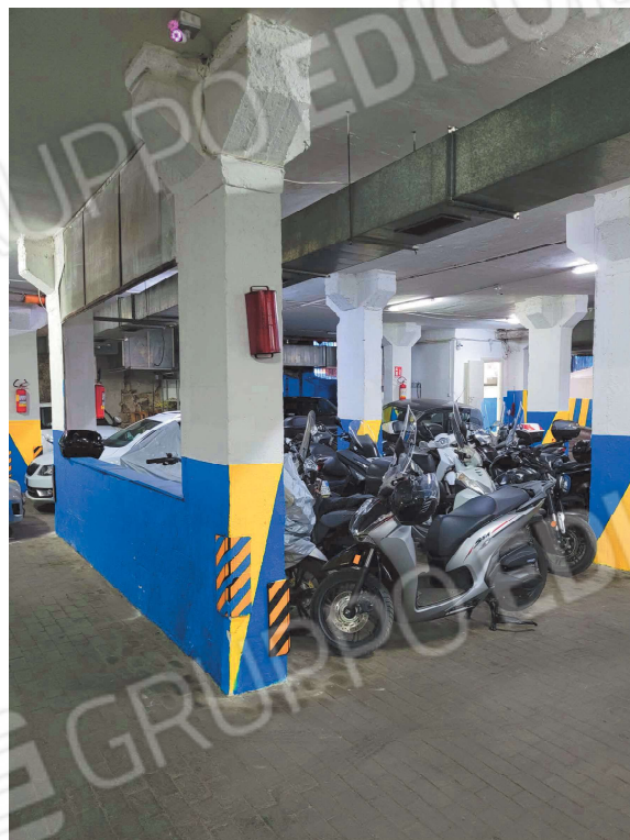
Vista locale garage
