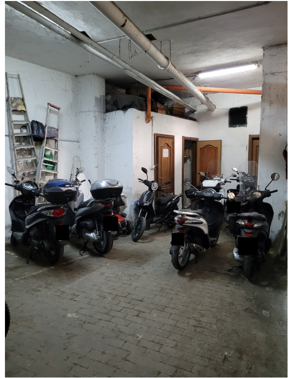
Vista locale garage
