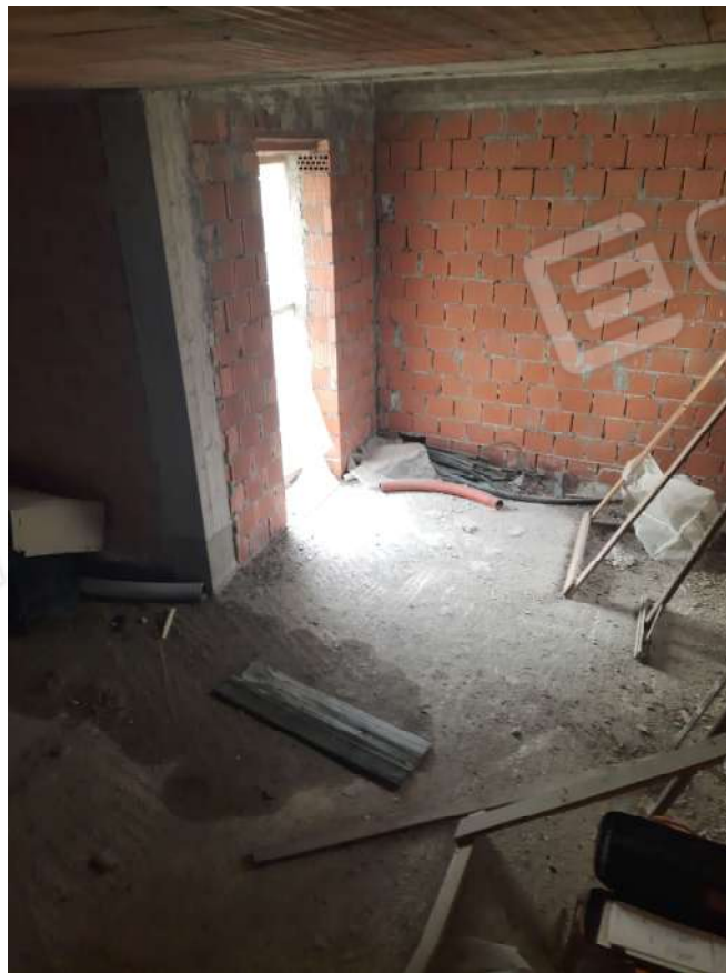
7- VISTA PIANO TERRA
