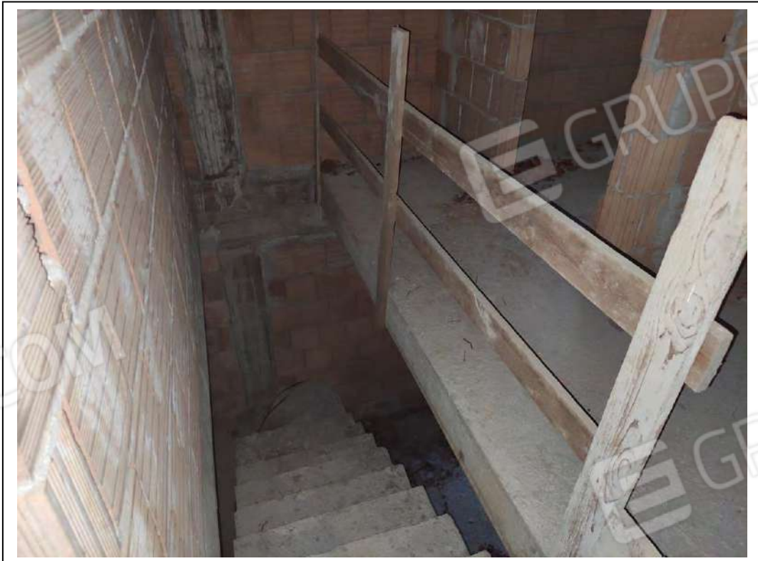
FOTO 12 – Sub. 502 – Piano Terreno
