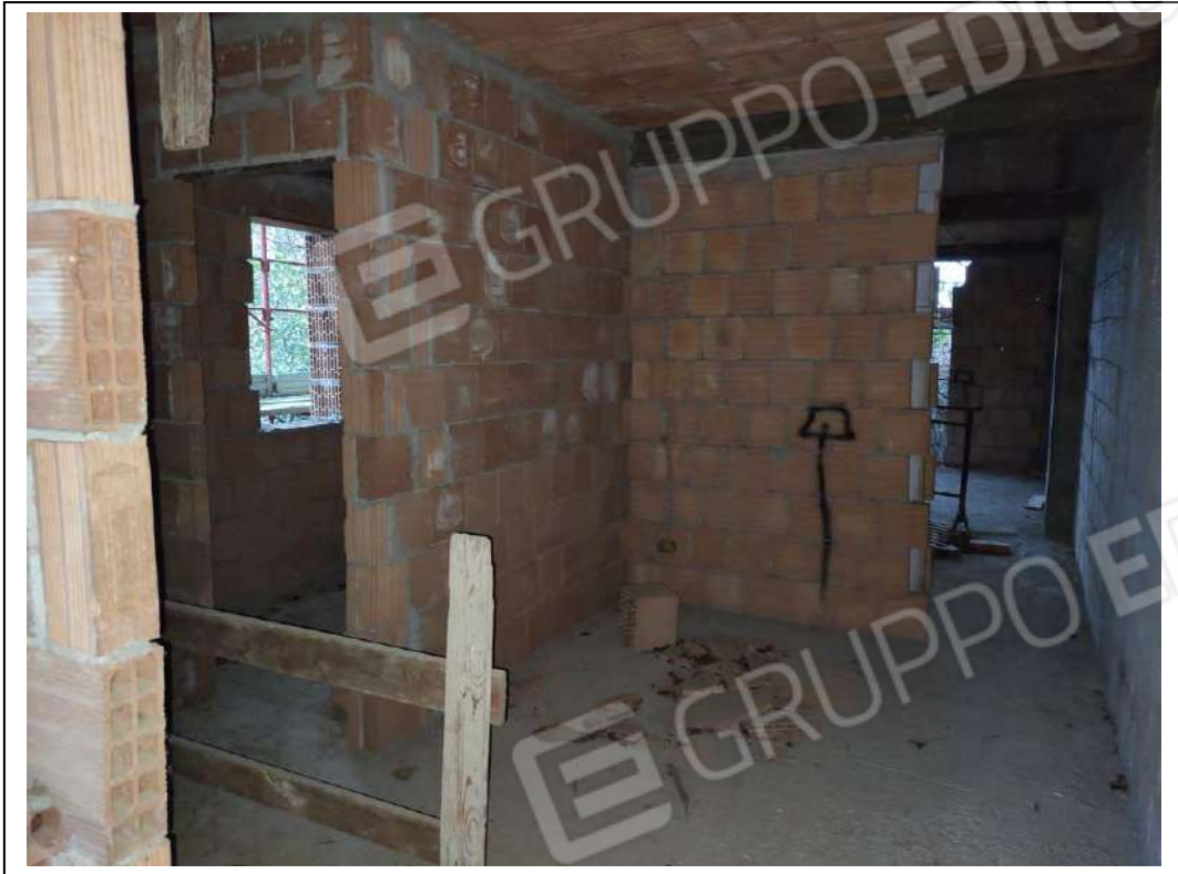
FOTO 11 – Sub. 502 – Piano Terreno
