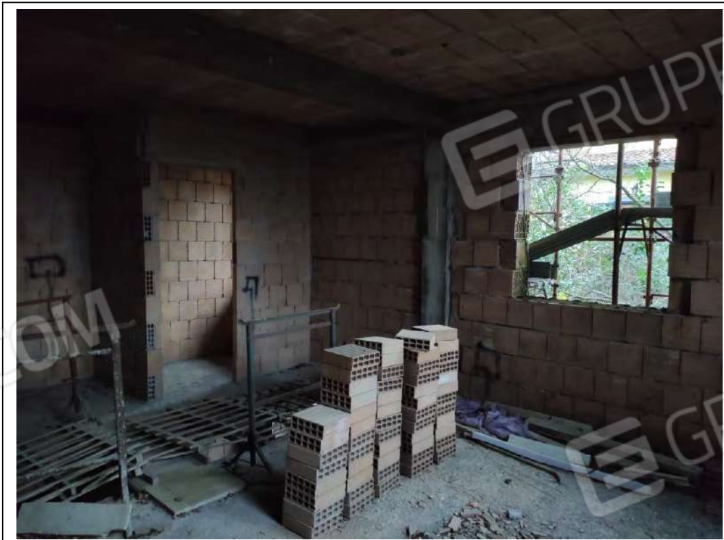
FOTO 14 – Sub. 504 – Piano Terreno
