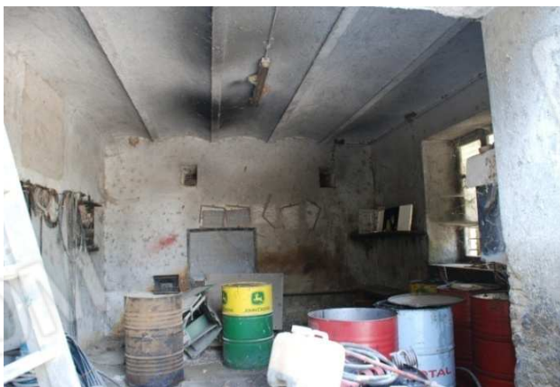
Piano S/2 - locale officina 1
