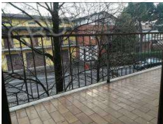
All. 51 – Balcone 1° Piano sub. 8
