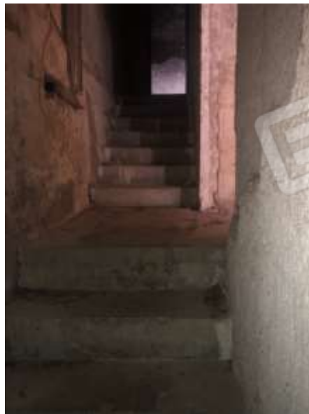
Scala piano interrato
