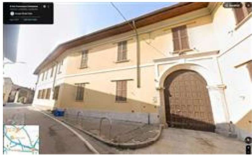
Vista da Google Street View
