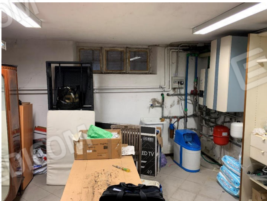
22 locale cantina piano seminterrato
