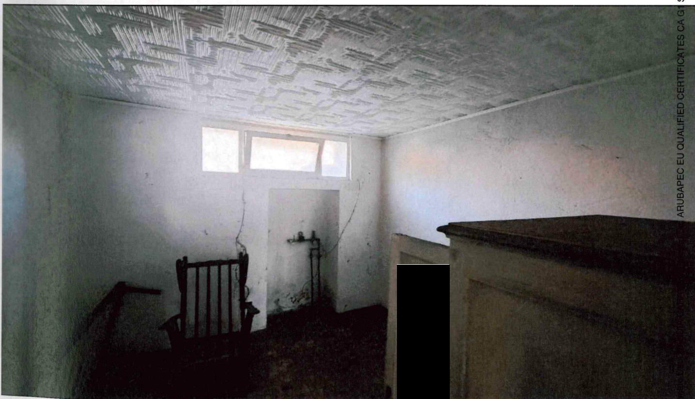
Piano seminterrato cantina
